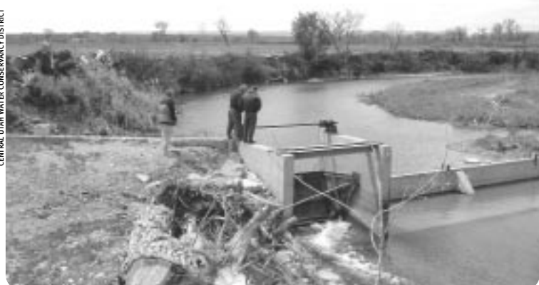
GENE SHAWCROFT OF THE CENTRAL UTAH WATER CONSERVANCY DISTRICT (RIGHT) JOINED DUCHESNE RIVER COMMISSIONER JOHN SWASEY (CENTER) AND U.S. FISH AND WILDLIFE SERVICE CREW LEADER TIM MODDE TO INSPECT THE MYTON TOWNSITE DIVERSION ON THE DUCHESNE RIVER. HISTORICALLY, THIS DIVERSION HAS FUNCTIONED AS A DRY DAM WITH DOWNSTREAM WATER NEEDS BEING SUPPLIED BY RETURN FLOWS. TO SUPPLY FLOWS FOR ENDANGERED FISH RECOVERY PURPOSES, THE DIVERSION WILL BE MODIFIED SO THAT FLOWS PASSED DOWNSTREAM CAN BE MEASURED AND ACCOUNTED FOR.
