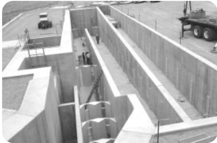
THE NEW FISH PASSAGE UNDER CONSTRUCTION IN MAY 2004.
