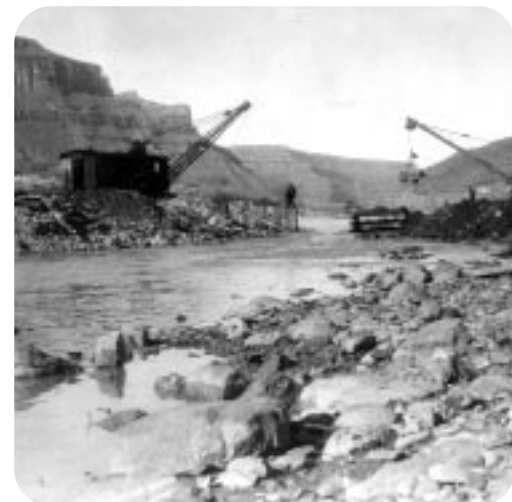
THE COLORADO RIVER AS IT WAS IN THE EARLY 1900S WHEN DAM CONSTRUCTION BEGAN.
